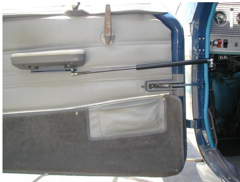
Figure 5. Installation Complete – Door Open
