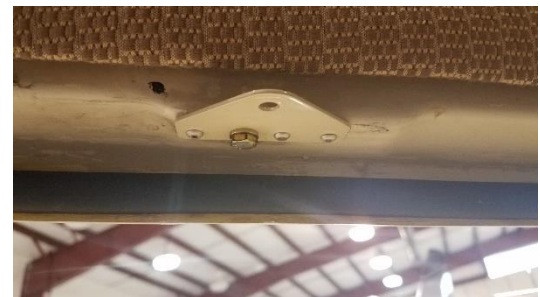
Figure 30. Door bracket attached
