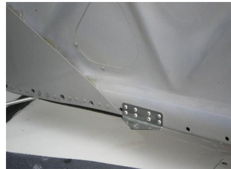
Figure 6. Door bracket installed
