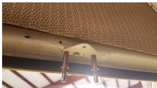
Figure 29. Drilling bracket to door
