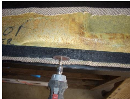
Figure 25. Slotting Interior Panel
