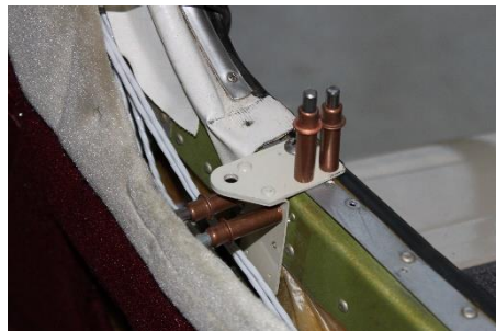
Figure 20. Airframe bracket utilized existing slide lock screw attachment
